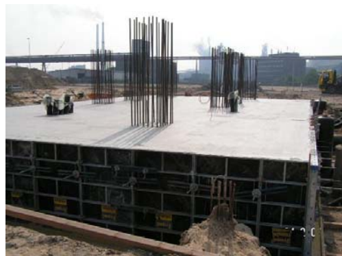
Pic. 3 Sleeve pipes after casting the concrete
