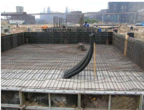
Pic. 2 Sleeve Pipe in the foundation later stage
