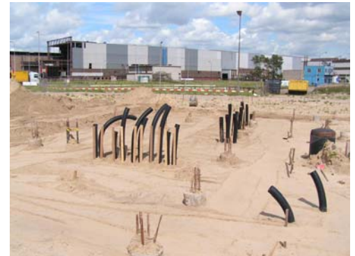
Pic. 1 Sleeve Pipe in the foundation
