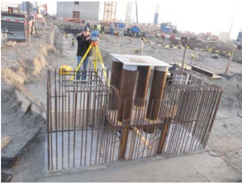
Pic.2.4 Sub construction fixed at an anchor box
