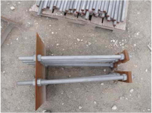
Pic. 1.1 Threaded anchor bolt with template and foot plate
