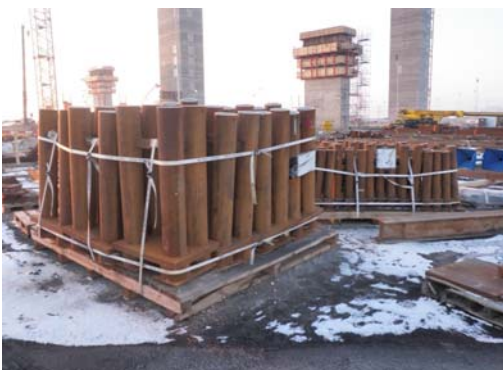
Pic.2.1 Anchors boxes at a pallet
