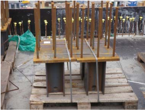
Pic. 3.1 Anchorplate with 9 rebar bolts
