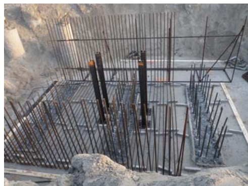
Pic.2.3 Sub-construction to carry the anchor box
